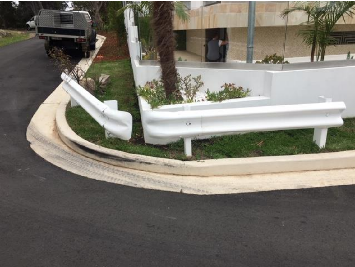
Pic 5- Bend at Woodlands Ave
