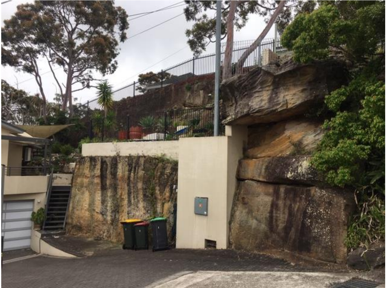
Pic 7- Drop at Intersection of Woodlands Ave and Taylor Ave
